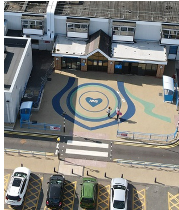
Aerial View of Hospital
