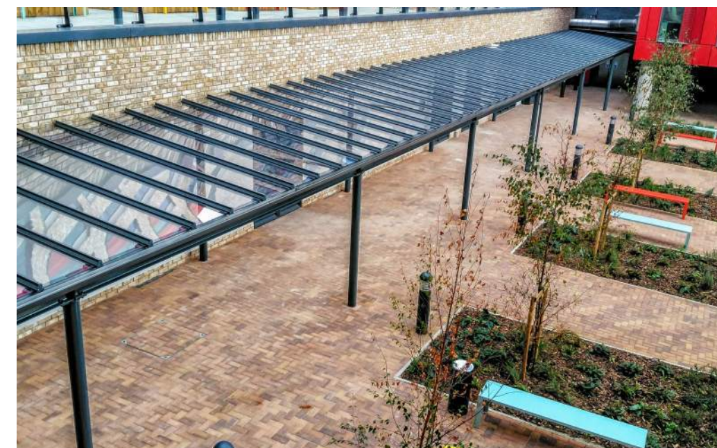
Project Example: Covered Walkway
