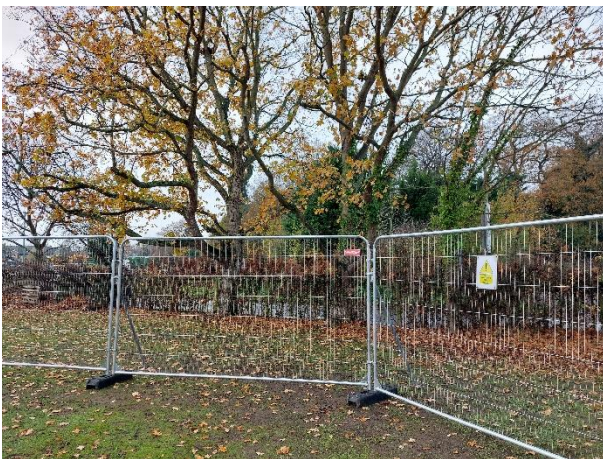
Photo 5: Heras fencing with base plate & sign.
