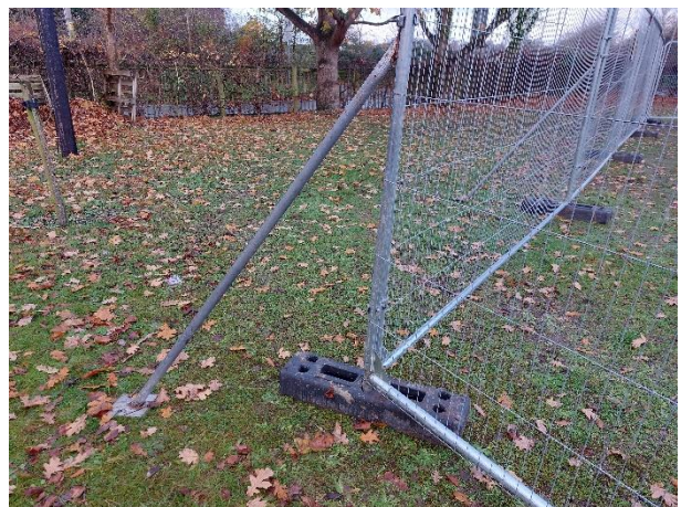
Photo 6: Block plate and stabiliser strut (pinned)
